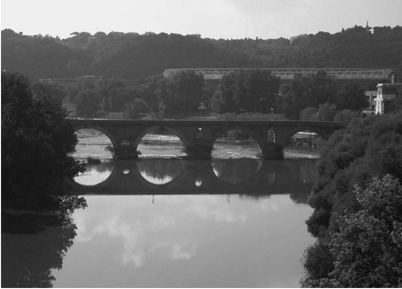
FIGURE 9. The Milvian Bridge, Rome, Via Flaminia. The superstructure of the bridge was rebuilt after its destruction in 1849, but its original piers remain. Photo by N. Lenski.
